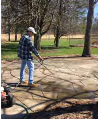
Clint Rossiter power washes the Sposeep Outdoor Chapel.
