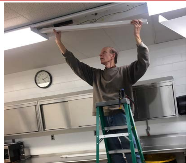
Maintenance Chief Clint Rossiter replaces the light fixture in the kitchen, the latest to be changed to LED at the Temple. Not only does the fixture provide brighter light, but the LEDs are more energy efficient and cost effective. We've also updated all the fixtures in the hallway by the Rabbi's office and the kitchen hallway.
